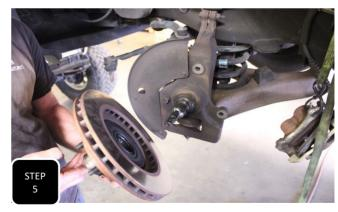
**Step 5** Remove the castle washer along with the nut and outer wheel bearing and then remove the brake rotor.
