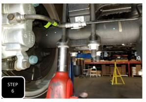
**Step 6** Once cut to length, install the U-bolts with the factory U-bolt plate and snug down. You will want to then loosen the U-bolts on the other side to allow the axle to rotate, and then fully tighten and torque the U-bolts to 140 ft/lbs. Next, install the block on the other side and torque down the U-bolts.
