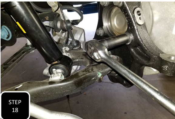
Step 18 Install the wheel bearing along with the factory dust shield using the factory bolts and tighten to 40 ft/lbs.
