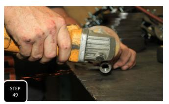
**Step 49** Remove the outer tie rod from the inner tie rod and mark a line 1/2" from the end of the threaded hole and cut this 1/2" section off. **NOTE: MAKE SURE YOUR CUT IS STRAIGHT SO THAT THE JAM NUT TIGHTENS UP PROPERLY.**
