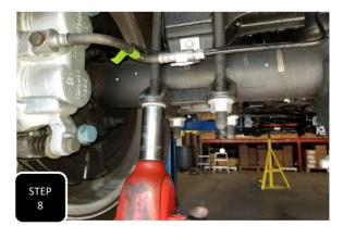
**Step 8** Once cut to length, install the U-bolts with the factory U-bolt plate and snug down. You will want to then loosen the U-bolts on the other side to allow the axle to rotate, and then fully tighten and torque the U-bolts to 140 ft/lbs. Next, install the block on the other side and torque down the U-bolts.
