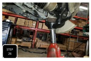
**Step 26** Locate the new, longer steering knuckles and install them on their designated side with the steering arm facing the front of the truck and the caliper mounting ears facing the rear of the truck. Use the factory hardware and torque to factory specs.
